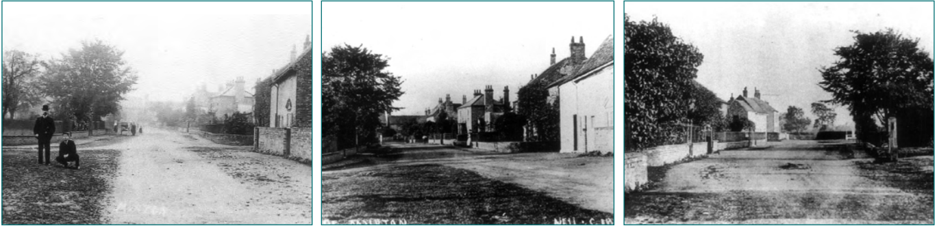
Views of Murton main street c.1900
