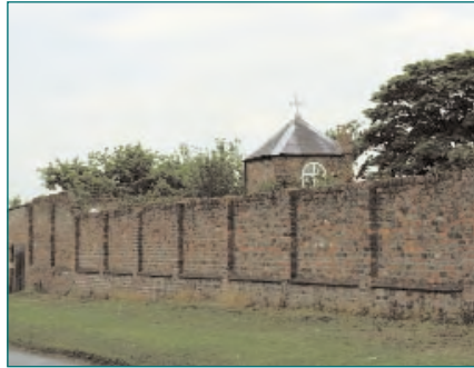
The wall and gazebo
